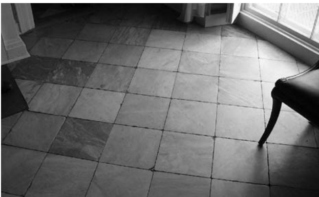
Figure V.5. Marble Floor Tiles in the Central Hall of the Gore Mansion House.
